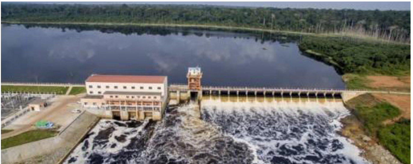
The Mékin Dam was finally commissioned by the Cameroonian government in May 2019. Source: businessincameroon.com
