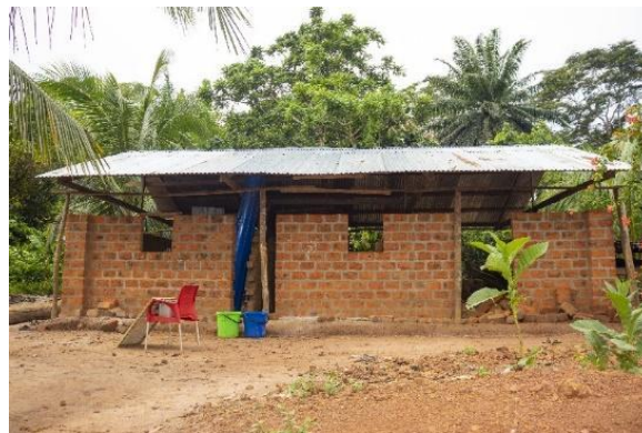
A house under construction
